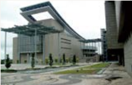
澳門文化中心綜合劇院 | Centro Cultural de Macau - Grande Auditório | Macao Cultural Centre Grand Auditorium 澳門冼星海大馬路文化中心 Avenida Xian Xing Hai S/N, NAPE, Centro Cultural de Macau
